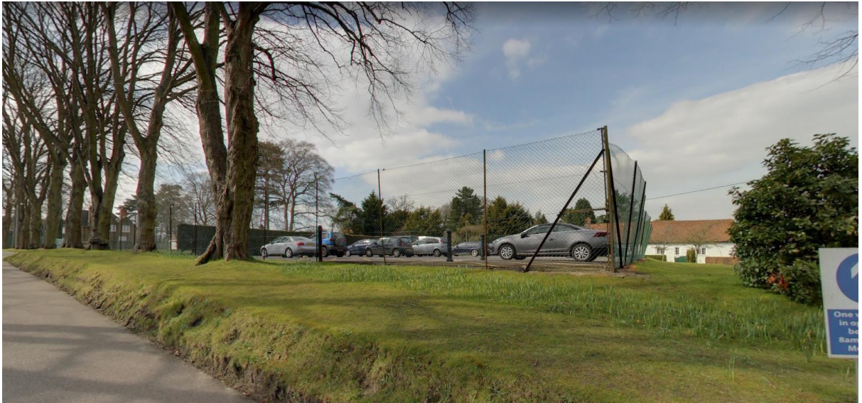
View of site looking west from Dauntseys School drive © Google
